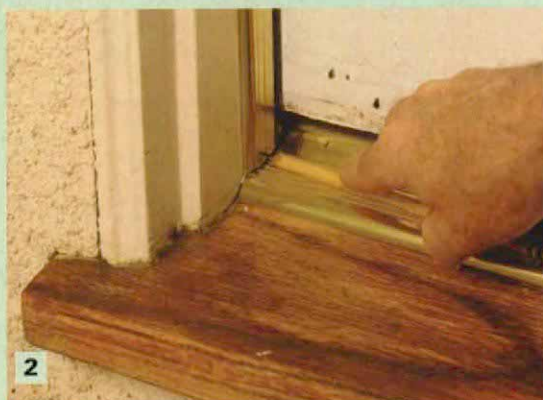
2 Scribe the legs to match the threshold. Weatherstripping on the side jambs usually lands on the sloped portion of the threshold, which means you will need to scribe the pieces to get a tight fit.
