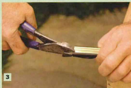
3 Crimp the ends to freeze the bulb. The vinyl or silicone bulb—the part that actually seals the door—will slide unless the metal is crimped at the ends.
