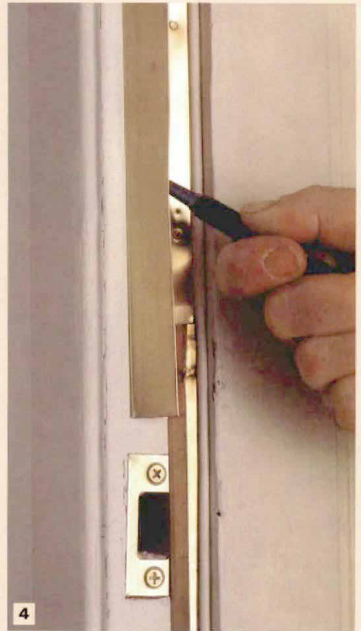
4 Use a nail set to adjust the strip. For large gaps, sliding a nail set into the crease will force out the flap. To press it back in again, slide the heel of the nail set against the flap.
